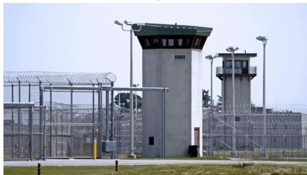
Tecogen was awarded a contract worth $1.4 million to install CHP units at a federal prison in New York.
