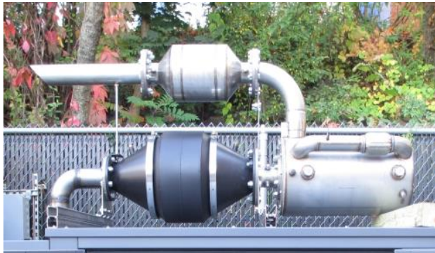
The Ultra Emissions System mounted to a CHP unit. The Ultra is designed to deliver simple, cost-effective solutions for natural gas engines to meet stringent emissions standards.
