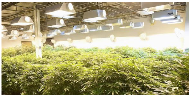
Intense lightning and space conditioning needed in indoor cannabis growing facilities place a heavy burden on most electric supply services.
