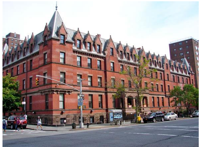
A nursing home in Brooklyn, New York will soon enjoy all the benefits of Tecogen's 375 kW microgrid cogeneration system (Image for illustration purposes only).
