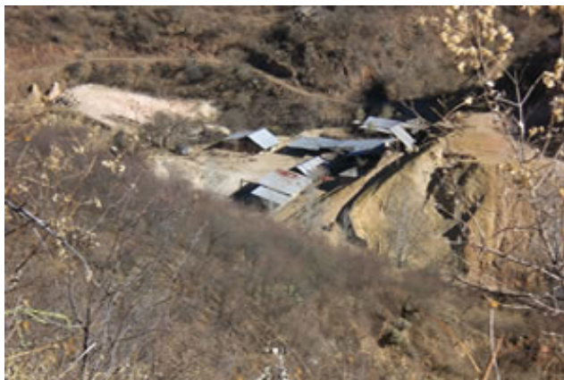
The actual Dios Padre open pit mill site. Note on the right the ore stockpile and old constructions of previous owners.
