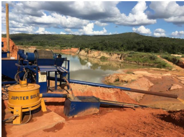
Jupiter Gold's modular recovery plant for gold.
