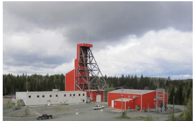
Part of the Francoeur Mine surface infrastructure.
