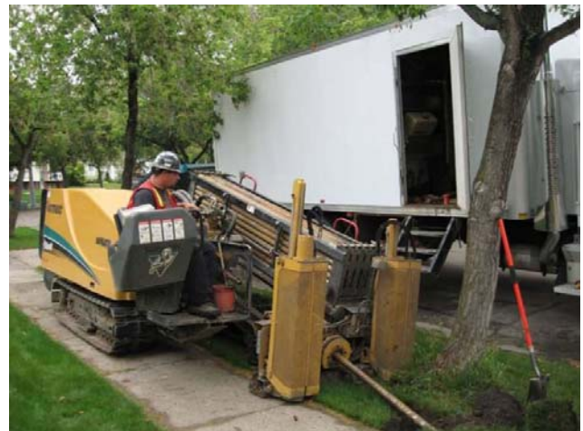
Directional drilling activities from Enterprise Oilfield.
