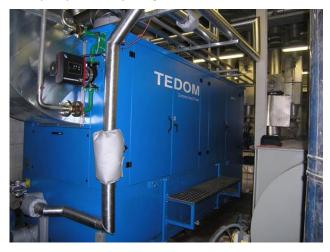
The 331kW TEDOM CHP unit at The Dome leisure center in Doncaster, UK will produce up to 1,848,470 kW of electricity and 2,038,343 kW of heat per annum, while saving up to 667 tonnes of carbon dioxide (CO2) each year - equivalent to taking 140 cars off the road.
