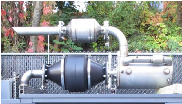
The Ultra Emissions System mounted on top of a CHP unit.
