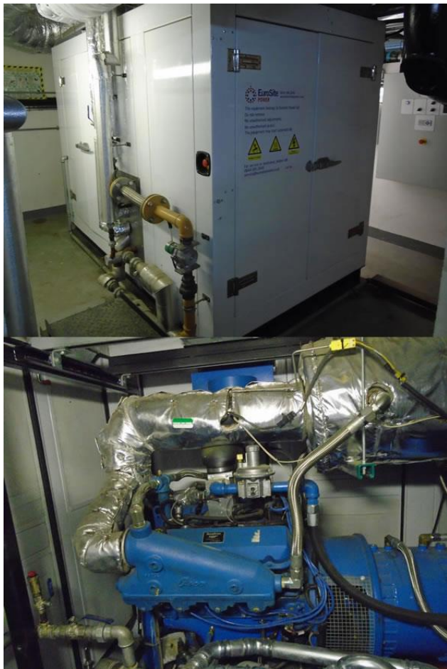
The Tennis & Health Club's CHP unit from the outside (top) and part of that unit's engine.
