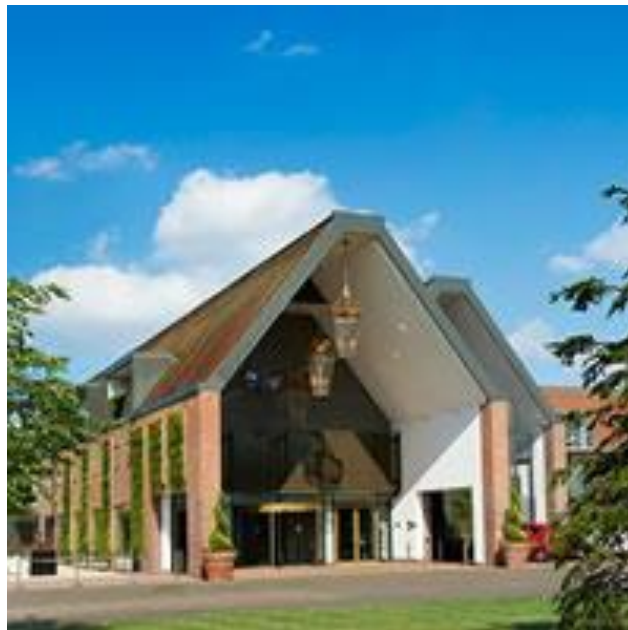
The Syon Park Waldorf Astoria in London was recently equipped with a 100kWe CHP unit.
