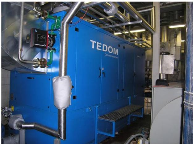
**The 331kW TEDOM CHP unit at The Dome leisure center in Doncaster, UK will produce up to 1,848,470 kW of electricity and 2,038,343 kW of heat per annum, while saving up to 667 tonnes of carbon dioxide (CO2) each year - equivalent to taking 140 cars off the road.**
