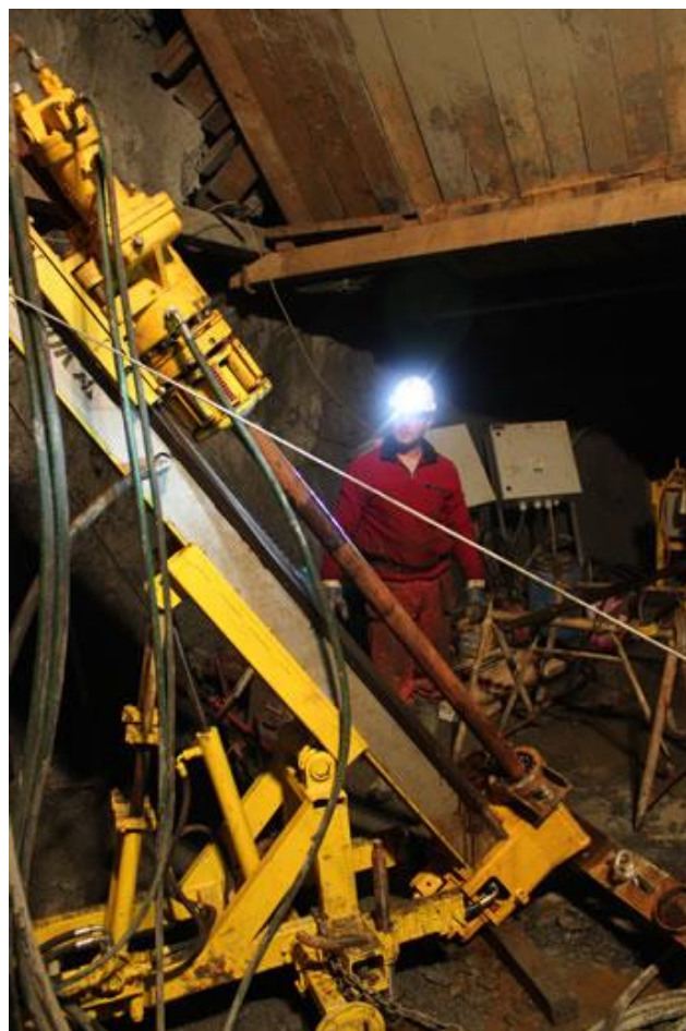
Underground drilling activities from Level 6, approximately 180 metres below surface, aiming at the Strieborná silver vein.
