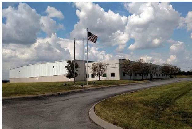
The new Spill Magic manufacturing and distribution center in Mt. Pleasant, Tennessee was purchased by Acme United (ACU) for approximately $6 million.
