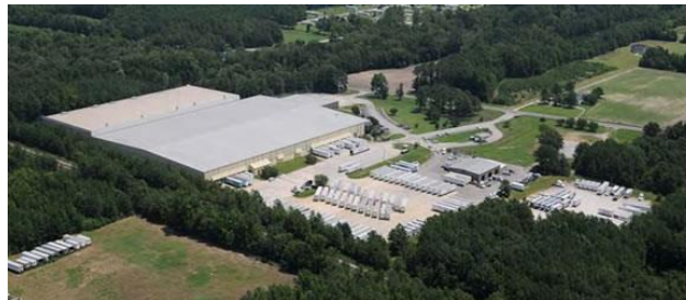
Acme's new manufacturing and distribution center in Rocky Mount, North Carolina has 40 foot ceilings and 27 bay doors.
