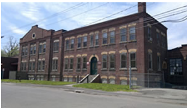
The Pac-Kit manufacturing plant in South Norwalk, Connecticut.
