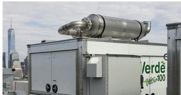
**The Ultra Emissions System mounted to a CHP unit. Hundreds of Ultras have been installed on cogeneration systems so far.**
