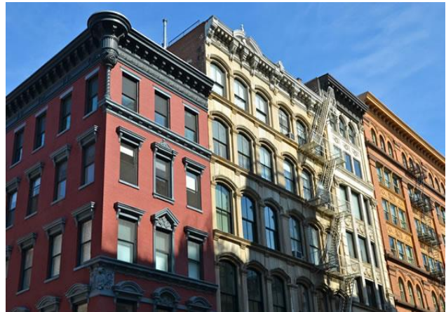
Seven 100 kW InVerde e+ CHPs will soon be installed in a large, multiunit residential complex in Manhattan, New York.
