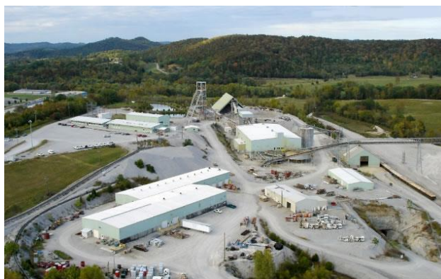
Located in the heart of Tennessee, the Nyrstar Tennessee Mines complex consists of six mines and two processing plants.
