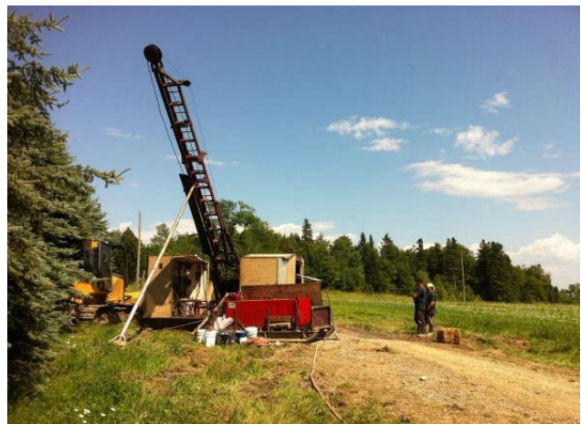
Drilling activity at the Woodstock Manganese property.
