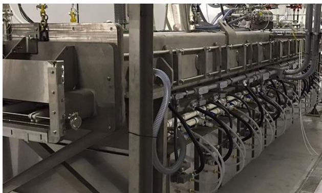
Part of a quantaREV dryer at EnWave's test facility.
