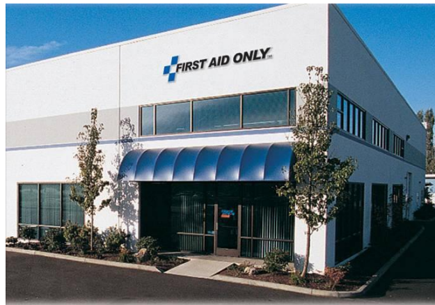
Acme paid $4 million for the First Aid Only facility, which is inexpensive, knowing that it was recently appraised at $6.25 million.
